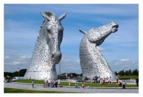
On 17<sup>th</sup> October we heard from Keith Jones about the origins of the Helix Park and the Kelpies. The Kelpies are nicknamed Duke & Baron. Built of structural steel with a stainless steel cladding they are 30 metres high and weigh 300 tonnes each. Construction began in June 2013, and was complete by October 2013 however the process of fabricating the steel was several years in the making.
